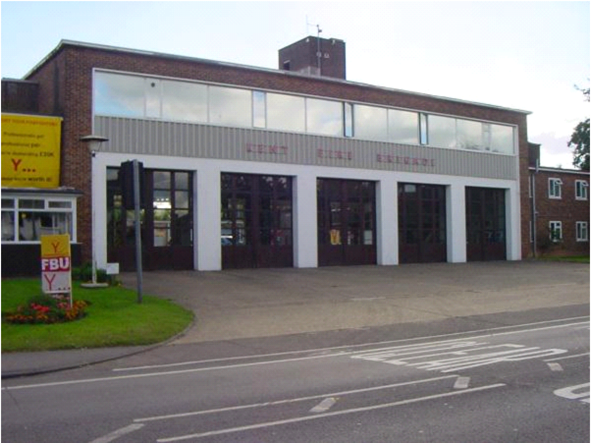
Maidstone Fire Station (60)
