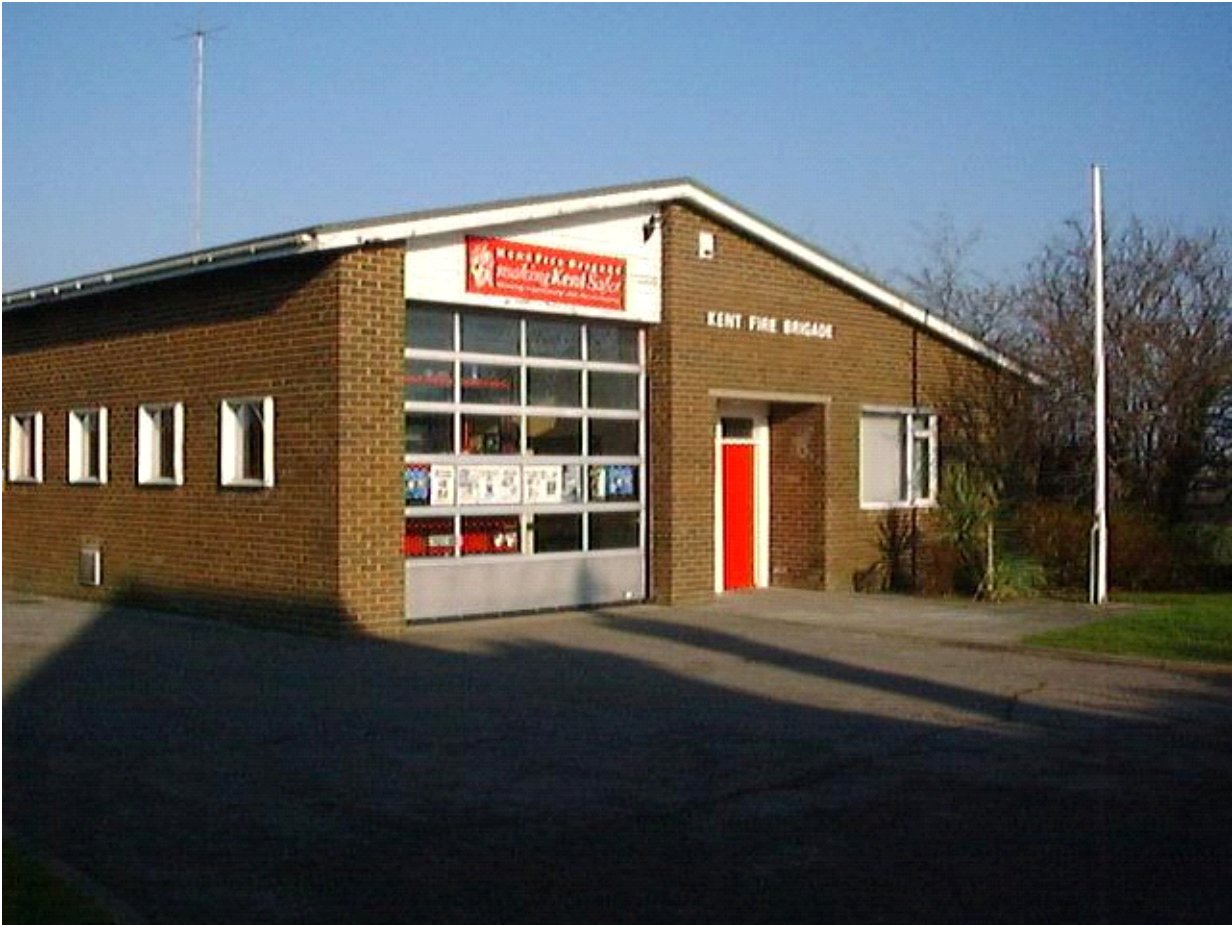
Wingham Fire Station (83)
